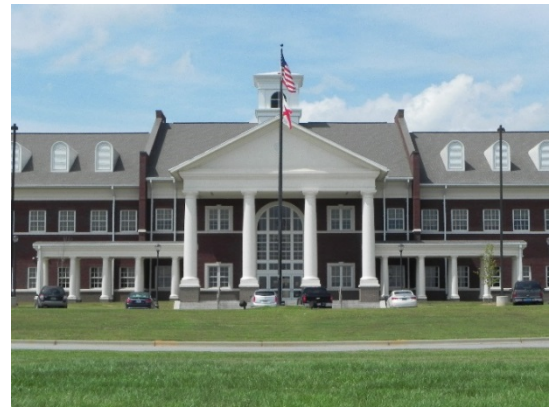
Central High School of Clay County, 2016.
