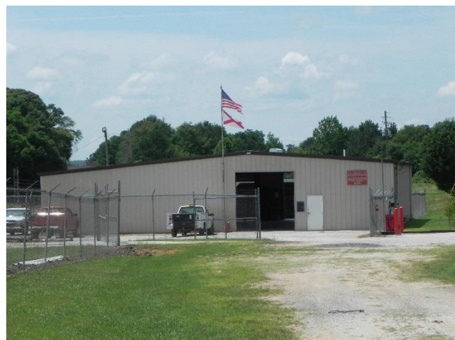
Lineville City Maintenance Building
