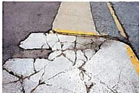
Non-compliant cracks
