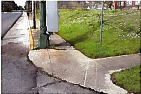
Obstruction with utility box
